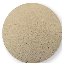
Carbonated concrete core after removal of soft chalky surface with scrubbing pad.
